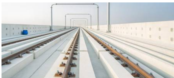
Рис. 1. Pre-cast PSC BLT Track Plinth
